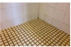
A number of wall tiles to the ensuite shower show of cracking and require replacing,
